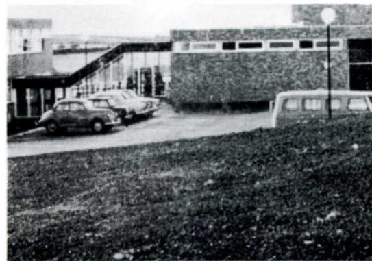
View of the Assembly Hall from the main car park
